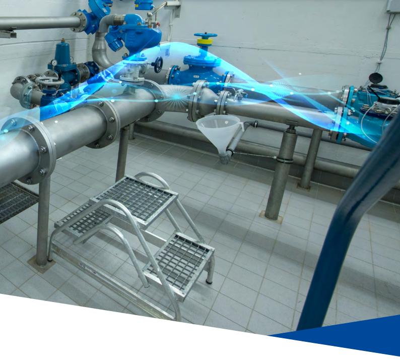
**Stationary ultrasonic measuring instruments** are ideally suited for metro logical monitoring of drinking water networks. The installation requires no intervention in the pipeline. This allows the simple and cost-effective installation of additional flow measuring points in an existing drinking water supply network.
